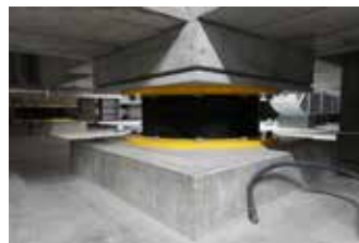
Seismic isolation rubber placed underground
